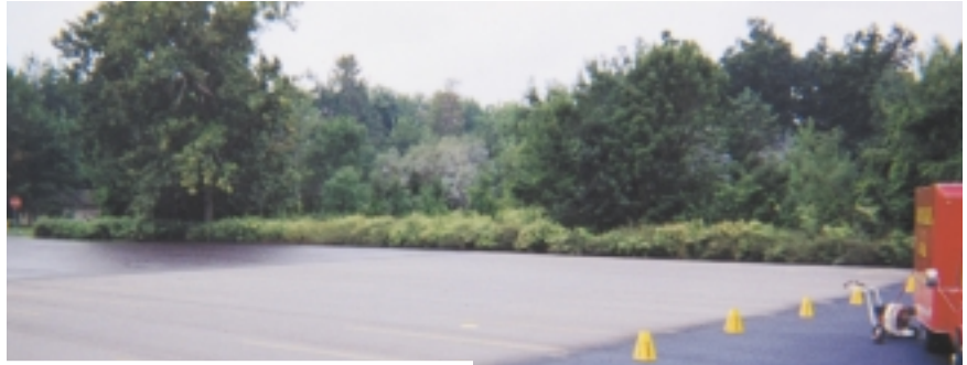
For Monroe Sealers of Rochester, Oscar Leon, holding hose, and Shawn Shales get the first coat of sealer down.
