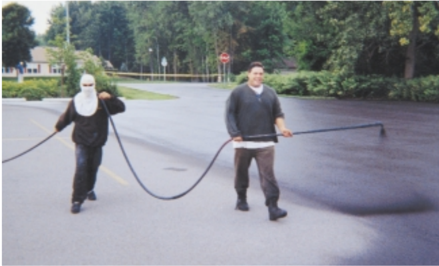
For Monroe Sealers of Rochester, Oscar Leon, holding hose, and Shawn Shales get the first coat of sealer down.
